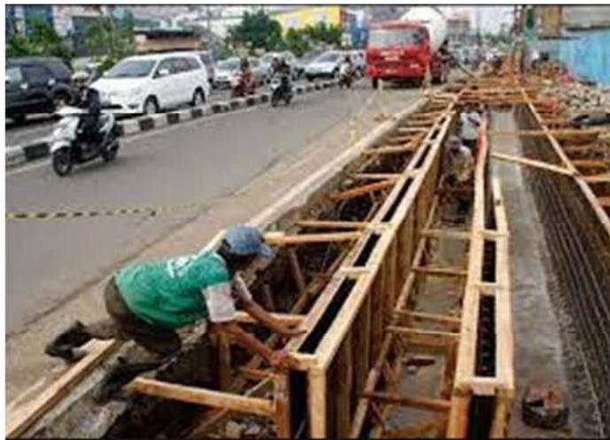
Figure 1. Drainage Costruction
